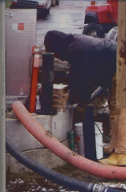
Karl Rice pumps and cleans a lift station that was being retrofitted with new components.
